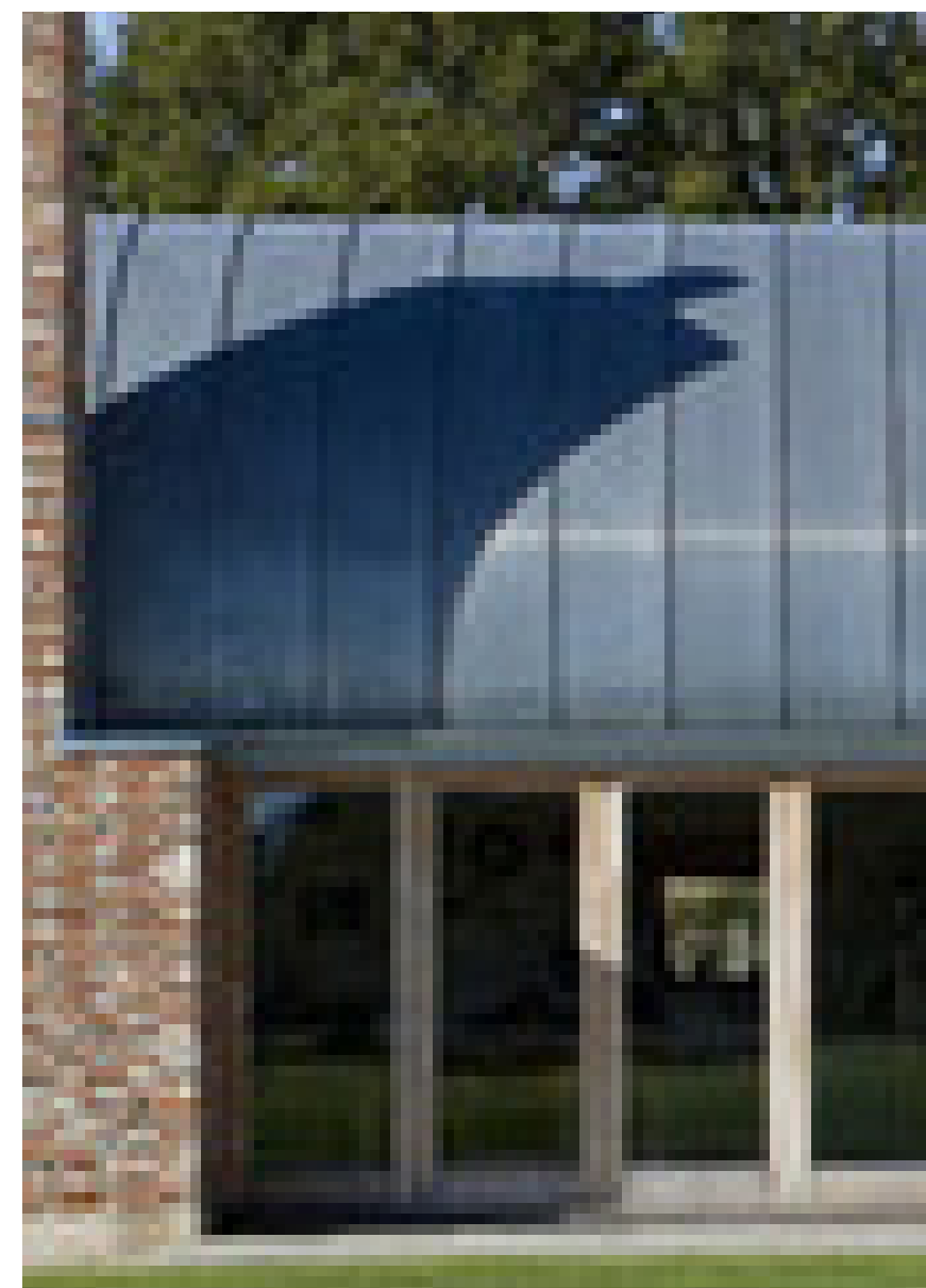
CURVED COPPER ROOF
