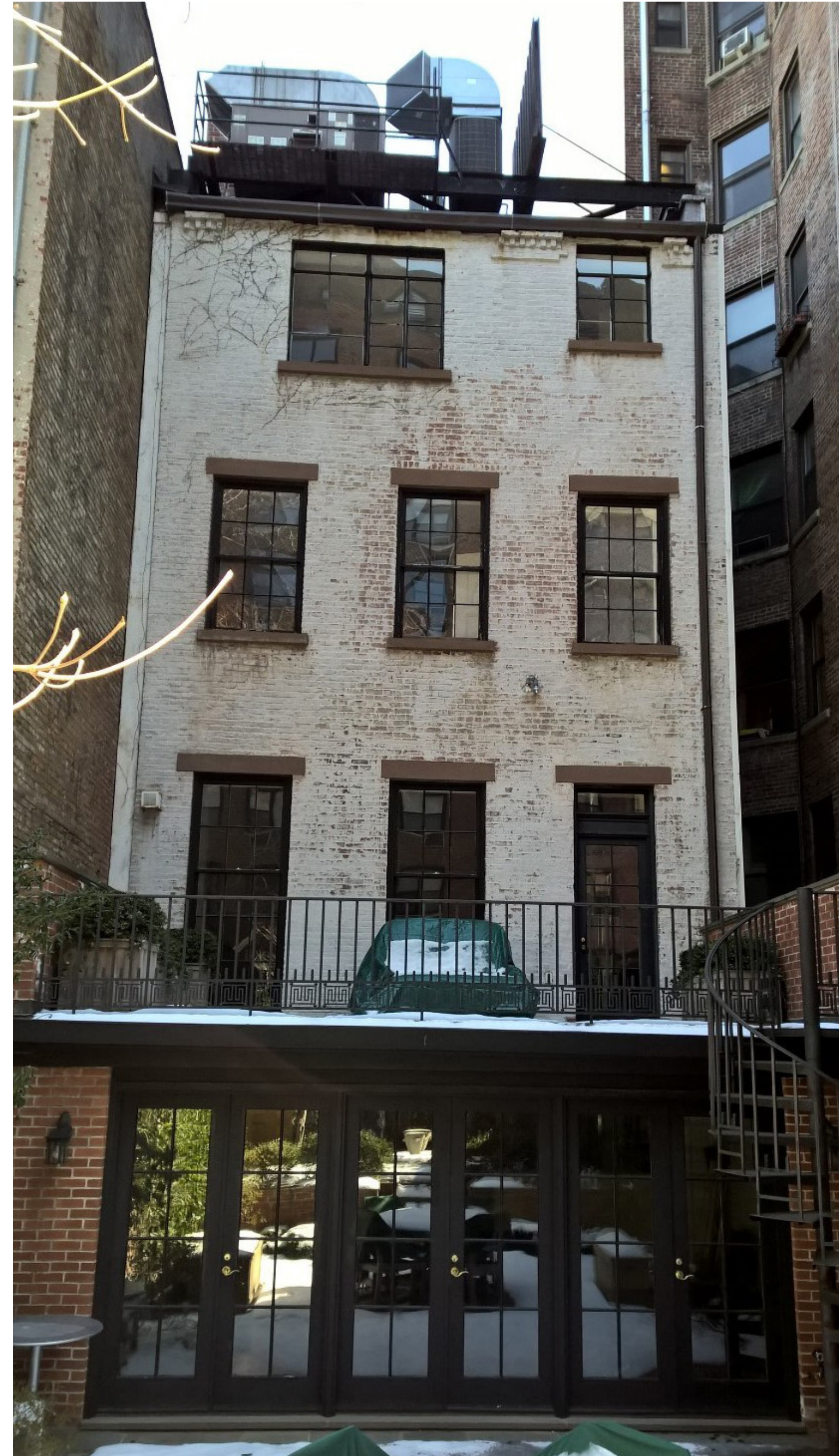
REAR FACADE (60 WEST 11TH STREET)
