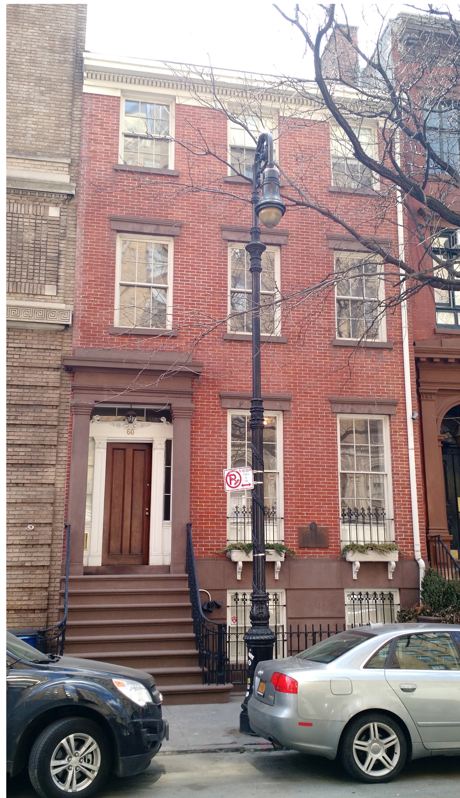
FRONT FACADE (60 WEST 11TH STREET)
